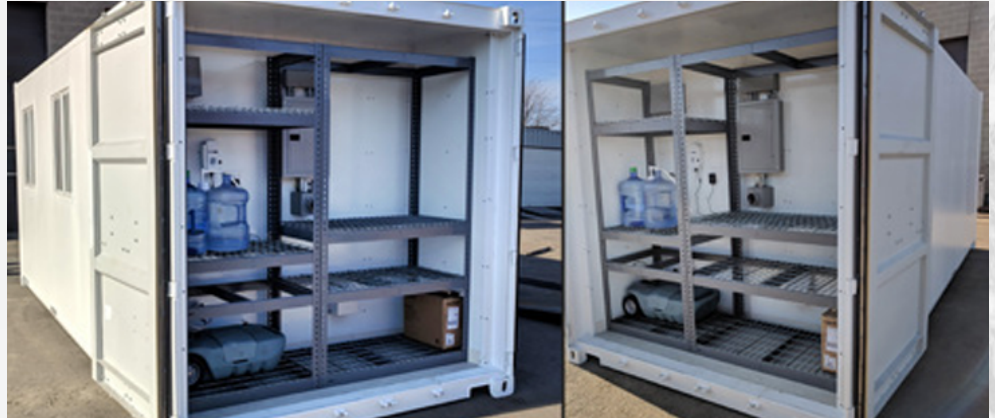
View from exterior at dedicated equipment room that is housed behind the cargo doors of the container. Customer wanted a solution that was highly secure, accessible, and functional. The modular shelving system can be (re)configured to accommodate various mechanical, electrical, plumbing, and communications equipment needs.
