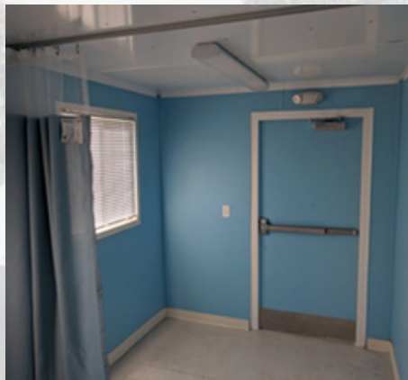
View from interior of exam room, looking toward entrance and waiting area. Push bar emergency exit device on door along with LED emergency lighting provides added safety.
