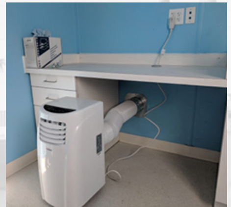
Portable air conditioner unit can easily be connected for use in high-ambient conditions while easily stowed when not in use.
